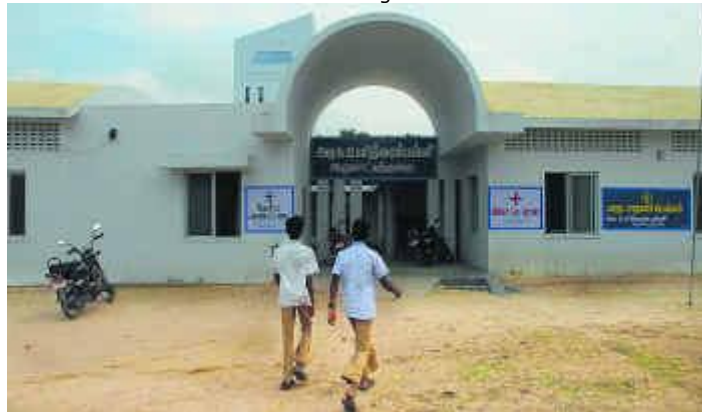
Learning as an enjoyable experience: The rebuilt school building.
